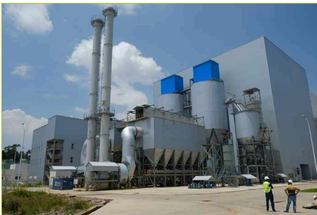
Figure 101 Reppie Waste-to-Energy facility
